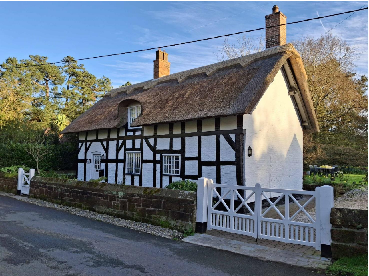
The Grade II Listed Old Post Office (looking good with its new ornamental block ridge)
