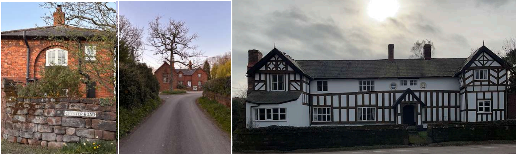
Left: Cross Cottage; the Village Hall and Old School Cottage; and Churton Hall. All are Grade II listed buildings.
