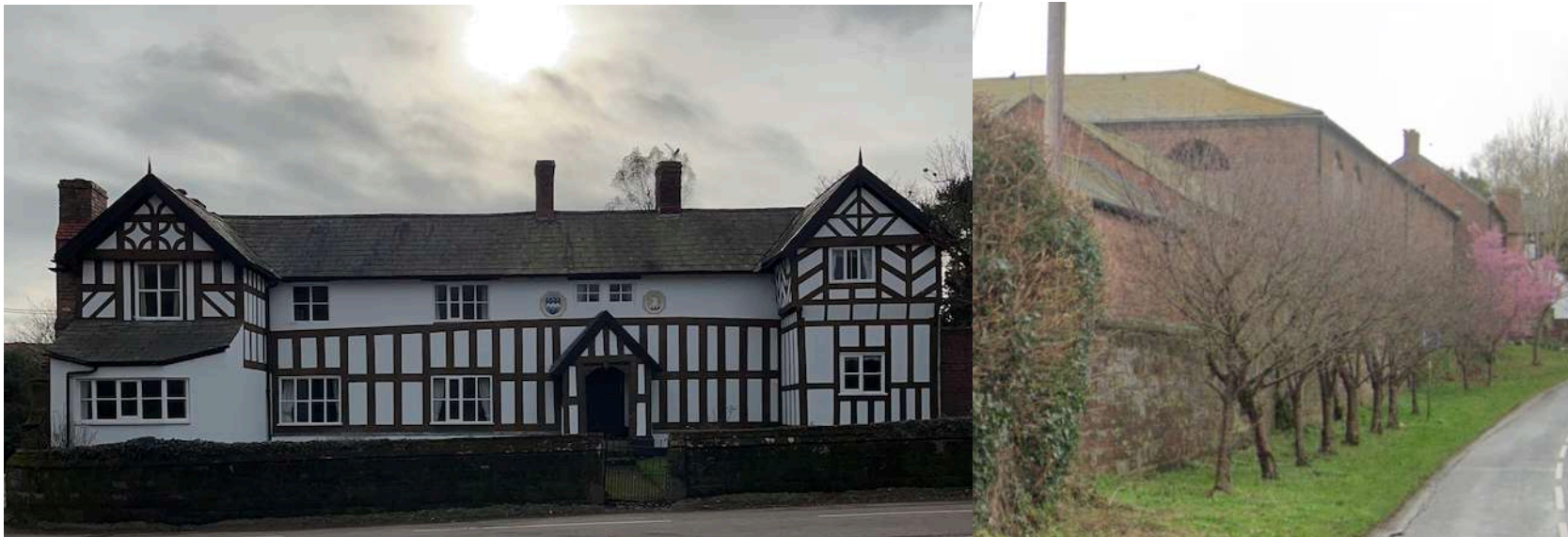
Left: Churton Hall Farm: Churton Hall (Grade II). Note the raising of the roof, probably undertaken in the 19 th century, with 19 th century casement windows; the smaller windows above the porch that replaced a dormer window; the off centre first floor window to the west wing; the central chimney stack is a late 19 th or early 20 th century addition the right chimney has been altered. The lateral chimney stack to the east gable has been truncated. The north west projecting gable perhaps retains some 19 th century vernacular revival chevrons to the first floor. Right: Churton Hall Farm outbuildings, seen looking west along Pump Lane, are curtilage listed buildings, a U-shaped range built in two phases.
