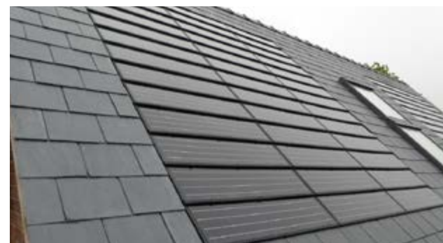
Figure 87: Contemporary solar panel design integrated in a traditional roofscape.
