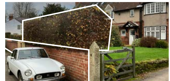
Figure 33: Sandstone walls, brick walls and hedges are common boundary features across Churton.
