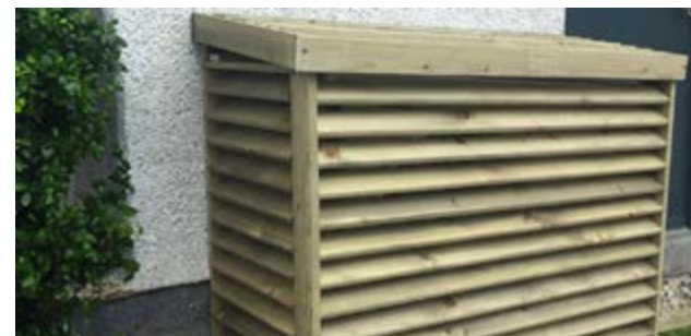
Figure 88: Air source heat pump housing covers the unit and harmonises with the parish's rural aesthetic.
