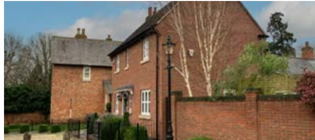
Figure 14: A new house in Rearsby, Leicestershire built from traditional red brick in Georgian proportions with good street interaction and active frontage.
