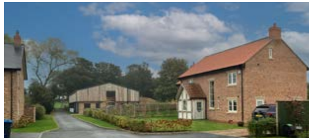
Figure 16: A new house in Helperby, North Yorkshire with modern window proportions but with red brick, red pantiles and a timber porch that reflect the local vernacular.
