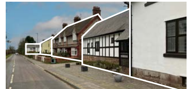
Figure 31: Chester Road highlights Churton's characteristic mix of building styles and materials.
