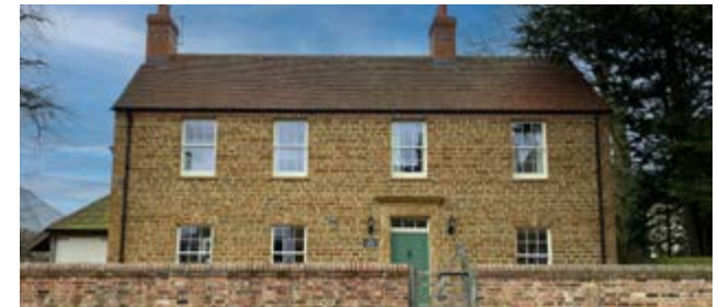
Figure 17: A new house in Great Bowden, Leicestershire built in local ironstone and incorporating the Georgian proportions of the surrounding historic buildings.
