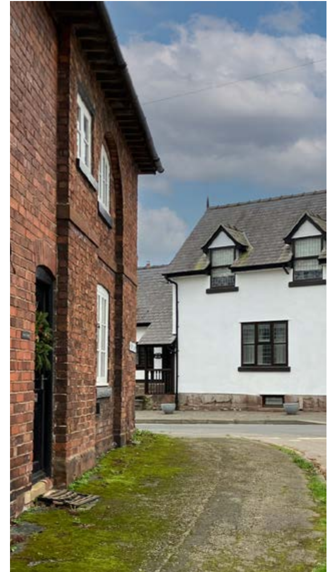
Figure 76: A positive corner interaction at the junction of Pump Lane and Chester Road whereby the building on the left addresses both streets.
