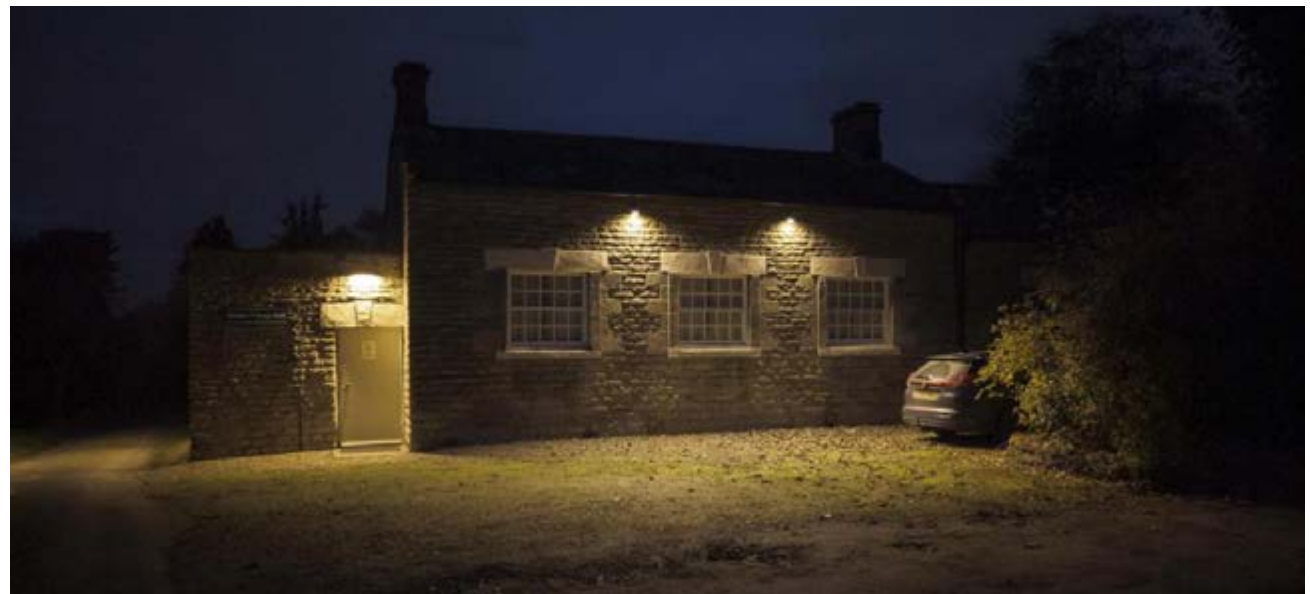
Figure 66: Dark sky compliant lighting at Bulmer Village Hall in Bulmer, North Yorkshire.
